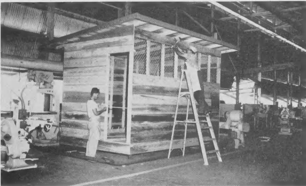
CARPENTER SHOP personnel finish the construction of a sled-type change house designed for field use. CARPENTER SHOP su personal ta completando construcion di un lugar pa cambia panja pa uso afor den Planta di un tipo movable.
